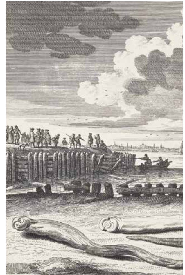
Abraham Zeeman, Naval shipworms affecting the dike campsheeting, 1731 (detail), 1731-1733.
